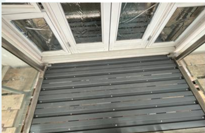
A Photo showing - Existing balcony decking removal and New decking installation works commenced and progressing
