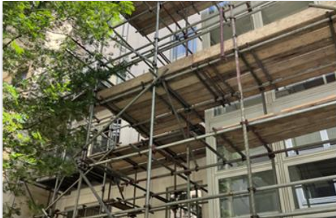
A Photo showing Phase 2 North Elevation - Scaffolding installation
