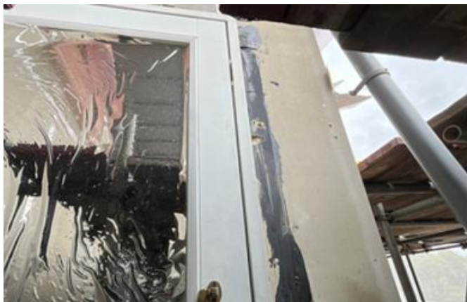
A Photo showing Phase 1 South Elevation - Existing cladding removal works progressing
