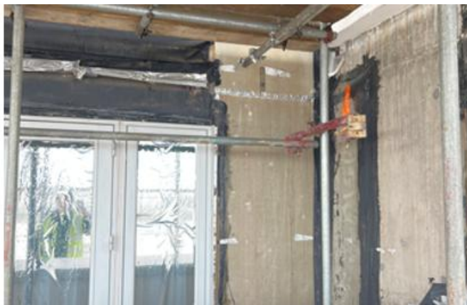
A Photo showing Phase 1 South Elevation - Existing cladding removal works progressing
